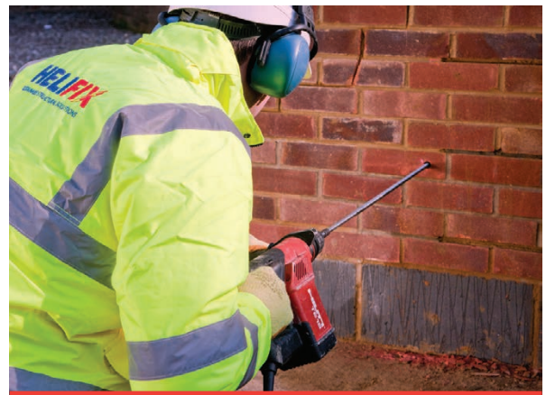
Drilling clearance hole for installing BowTie into joist end
