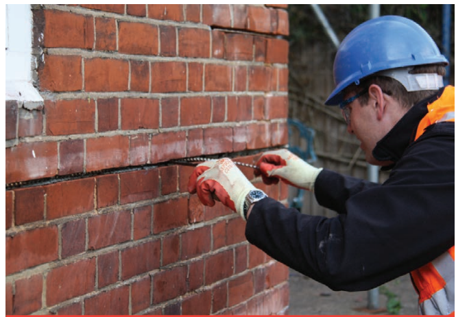
HeliBar is inserted into the HeliBond grout within the cut slot
