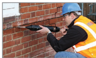
3. Using the Helifix Pointing Gun Kit, inject a bead of HeliBond along the back of the slot.
