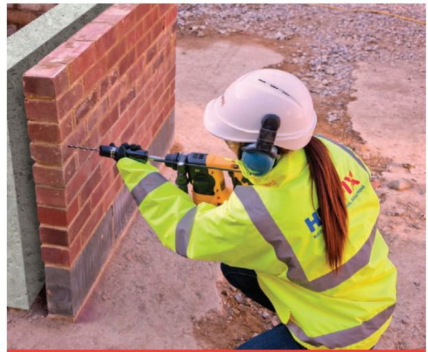
DryFix tie being power-driven into pilot hole
