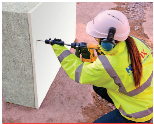
StuccoPin being power-driven into pilot hole
