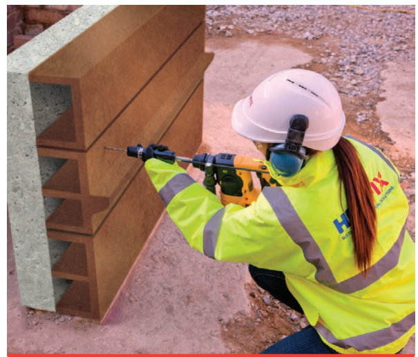
DryFix tie being power-driven into pilot hole
