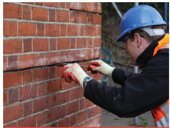
HeliBar is inserted into HeliBond grout within a cut slot
