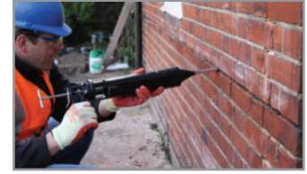
5. Insert a further bead of HeliBond over the exposed HeliBar, finishing 12mm from face and 'iron' firmly into the slot using the HeliBar Insertion Tool
