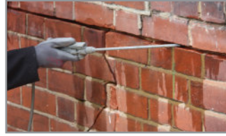
2. Clean out slots and flush with clean water and thoroughly soak the substrate within the slot
