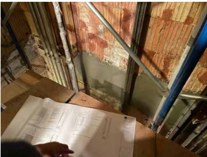
Surveying the shaft
